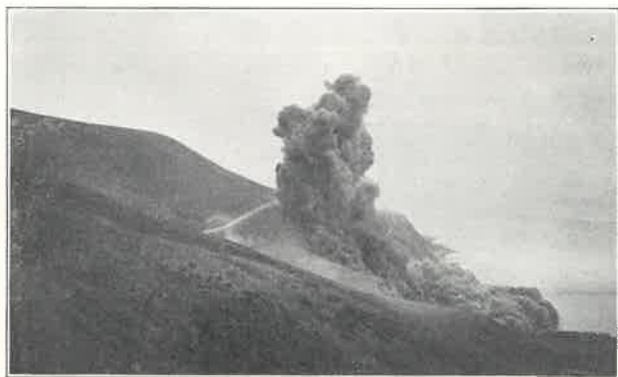
BLOWING UP THE "DOUGLAS CUT" FOR THE NEW SHORE HIGHWAY, OCTOBER 17TH, 1923
