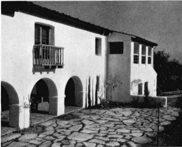
A FLAGGED OPEN PATIO AT THE GARD RESIDENCE Via Campesina, Malaga Cove
