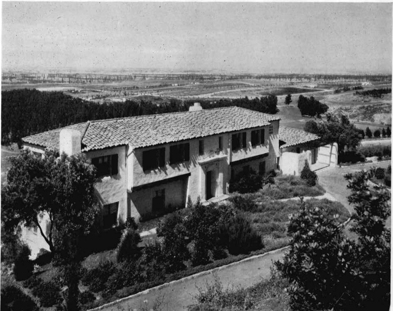
THIS HOME ON VIA HORQUILLA HAS A WIDE VIEW OVER THE GOLF COURSE TO THE NORTH
